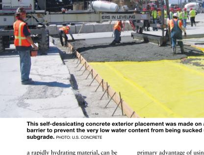
slab drying times are initially a little longer with a barrier but drying time is reduced by preventing ground moistrure from being added to the system. Without a vapor barrier, a slab on ground will never dry out.
