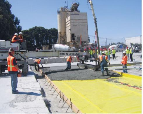
This self-dessicating concrete exterior placement was made on a vapor barrier to prevent the very low water content from being sucked up by the
