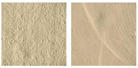
ICRI's CSP-2 (left) and CSP-3 (right) profiles shown are the most commonly specified surfaces for surface membrane systems. PHOTO: JOE NASVIK
