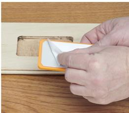
4) Remove the release paper covering the butyl seal on the Floor Sentry and apply the device so that the butyl seal bonds with the wood inside of the cavity. Afterward, proceed with the flooring installation as planned.
