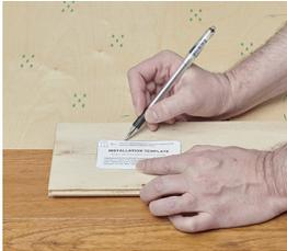
2) Use the included installation template card to outline a correctly sized space for the Floor Sentry device. The template card will also help you determine the correct depth that the cavity needs to be for optimal function. Refer to your Floor Sentry manual for details.
